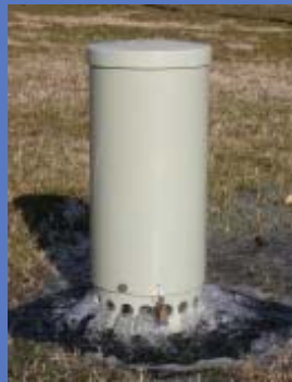
Eclipse #9400 Automatic Flusher (flushes to ground)
